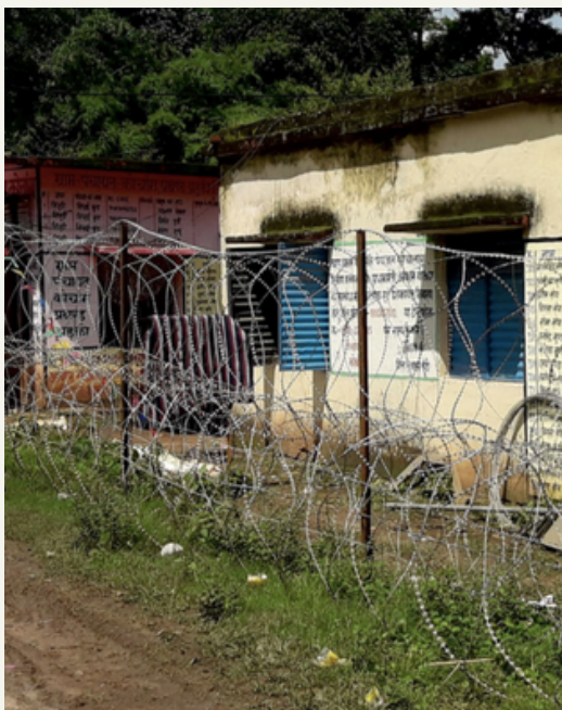
Occupation of Paramilitary Forces and barbed fencing at a Panchayat Building at Khunti, Jharkhand 2018 Photo: Puja
